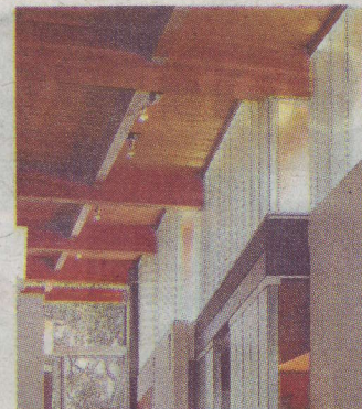
The high ceiling is remarkable for vertical steel beams, Douglas fir cross beams and channel glass windows.
